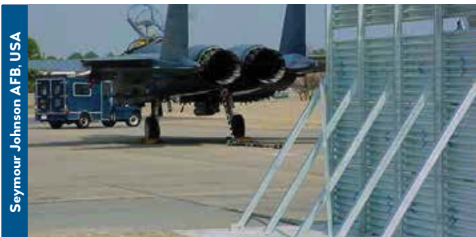
Deflectors rated for full power afterburner testing of fighter aircraft.
