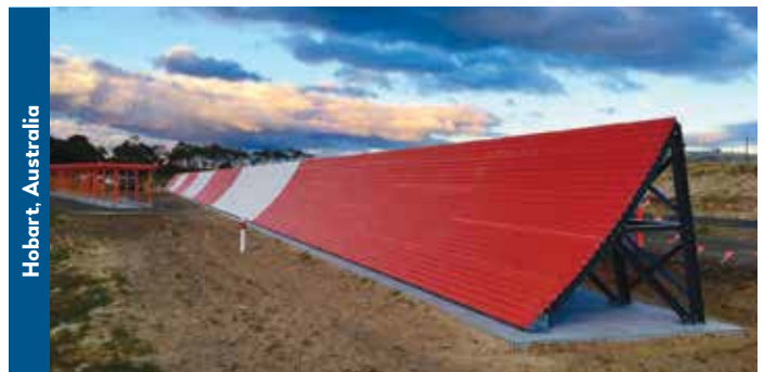
Fiberglass deflectors for use near NAVAIDs.
