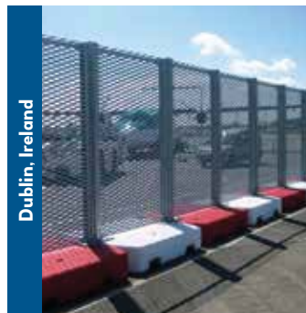
Expanded metal (mesh) deflectors for taxi-breakaway applications.
