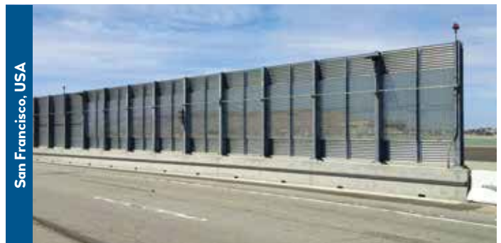
Vertical blast fence with both solid and mesh material.
