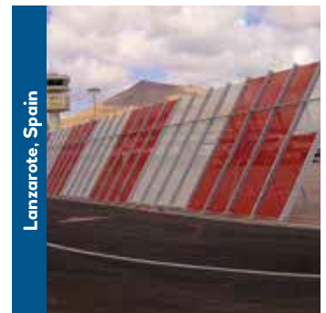
Expanded metal (mesh) deflectors for taxi-breakaway applications.
