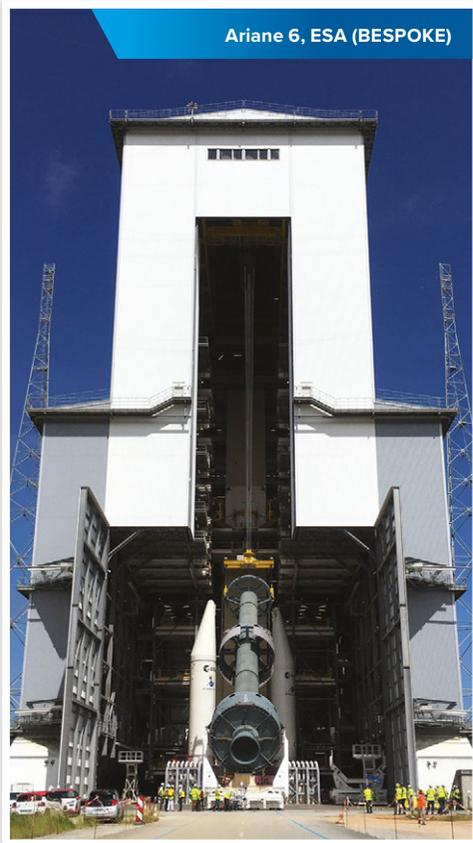
In collaboration with major architects and contractors Jewers offers a bespoke door design and specification service. Whether it is a 12 metre wide by 5 metre high sliding/folding door finished with a perforated aluminium sheet for a supermarket loading bay in Central London, or a 70-metre high double stable door to house Ariane-6 for the European Space Agency in French Guiana, Jewers do Bespoke.
