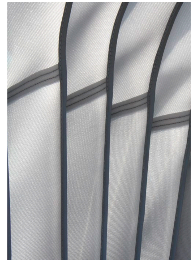
▲ Translucent folding bellows make the canopy airy and light
